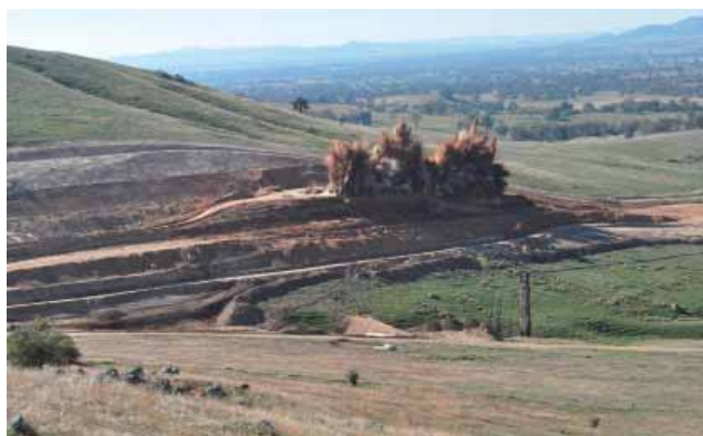
The first blast at the northern end of the Woomargama Bypass project, Hume Highway.
