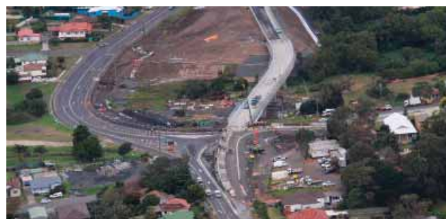
The Bulli intersection upgrade, Princes Highway.
