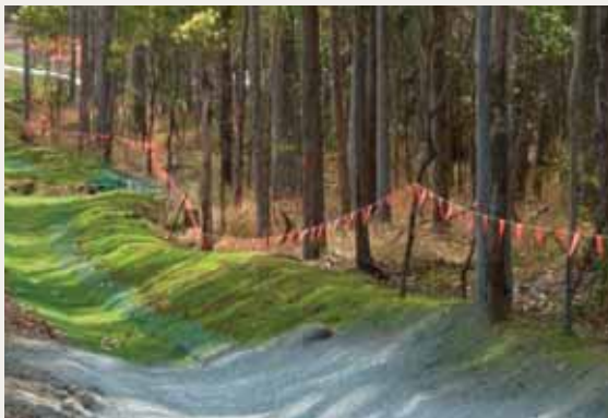
High visibility flagging protects vegetation on the Glenugie upgrade construction site.
