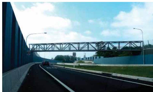
Northern Distributor extension in Wollongong, November 2009.
