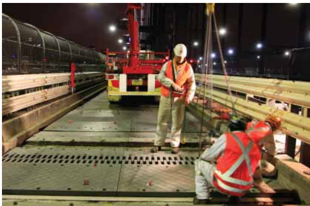
Night works on Sydney Harbour Bridge.
