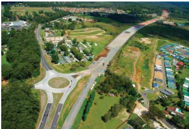
Aerial view of the Oxley Highway upgrade at Port Macquarie, to the west from Wrights Road roundabout.
