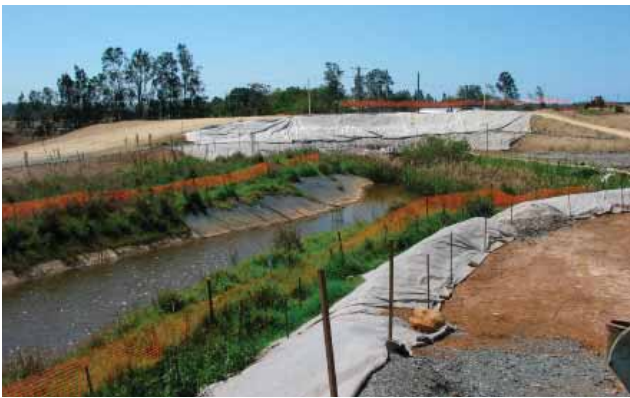
Stormwater controls minimise erosion on the Ballina Bypass construction site.
